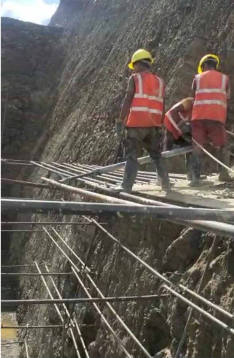
Anchoring for slope protection
